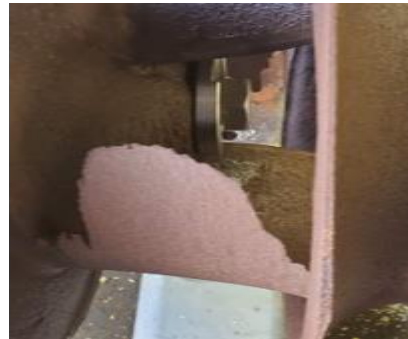
Abrasive damage to impeller vane
